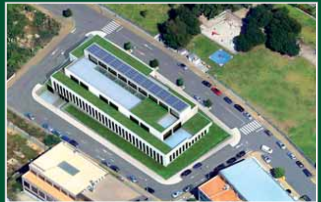
■ Project: Disashop Central Headquarters ■ Location: Rua Icaro, 2c-15479 Oleiros (A Coruña) ■ DIADEM® Partner: COMERCIAL PROJAR, S.A.
