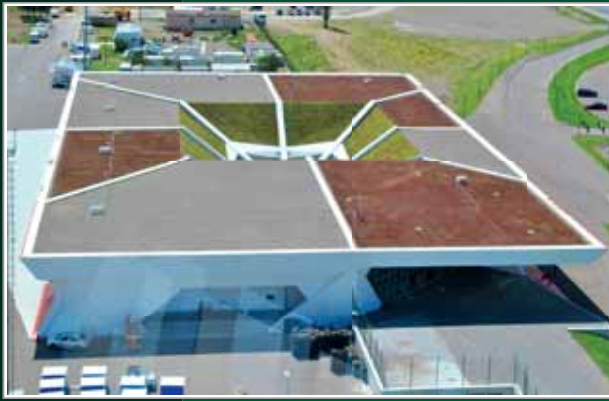
■ Project: Kopitnari Airport ■ Location: Kutaisi, Georgia ■ Architect: UNStudio; Amsterdam, NL ■ DIADEM® Partner: Hydroproof Kft, LTD Green House
